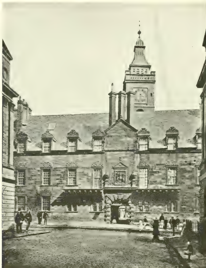
Front of Glasgow College in 1870. From a photograph by Messrs T. & R. Annan.
